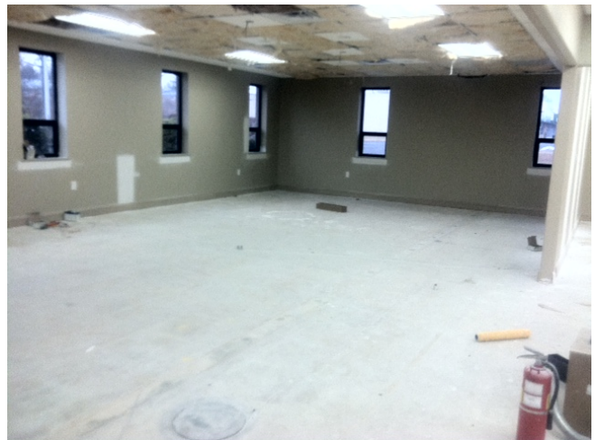
New Board/Conference Room
